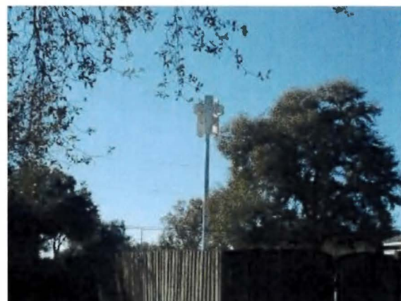
Street view from South Devonshire Lane
