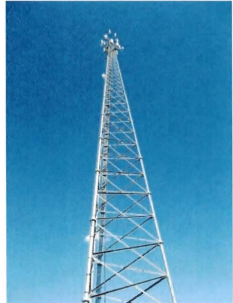
View of tower from the base compound
