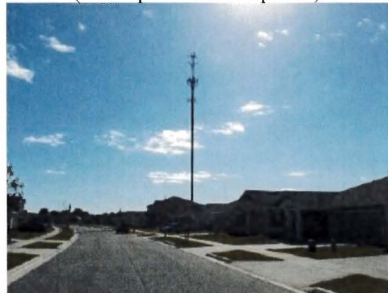
Tower views from South Andrea Circle
