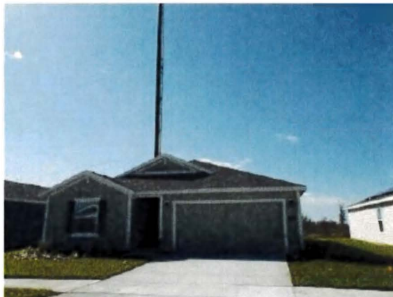
Tower views from South Andrea Circle
