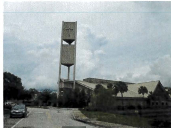
Street view of bell tower installation
