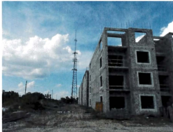
Azaela Park Rental Community under construction
