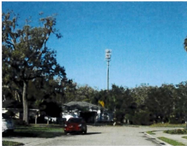
View of tower from front of property
