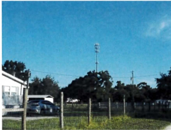
Lakewood Ranch, Sarasota County – Monopole Tower
